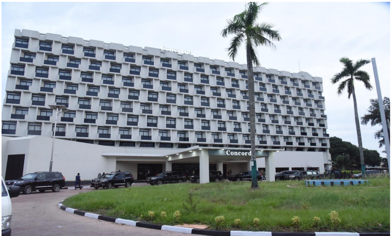
RECONSTRUCTED IMO CONCORD HOTEL
